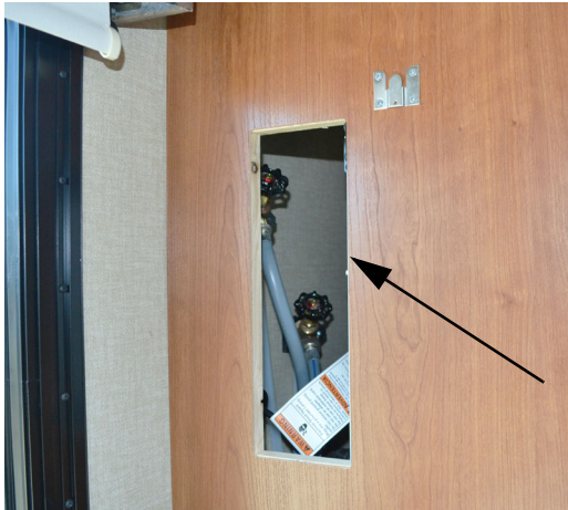
Water Supply Faucets (Located behind access panel rear of washer/ dryer) *Model 36H
