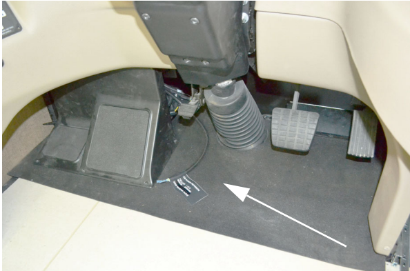
CB Power Wires -Typical View
