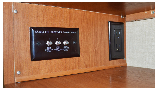
Interior Satellite Dish Connections (Located in the entertainment center cabinet) -Typical View
